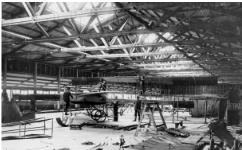
CFS Repair Shop January 1913
